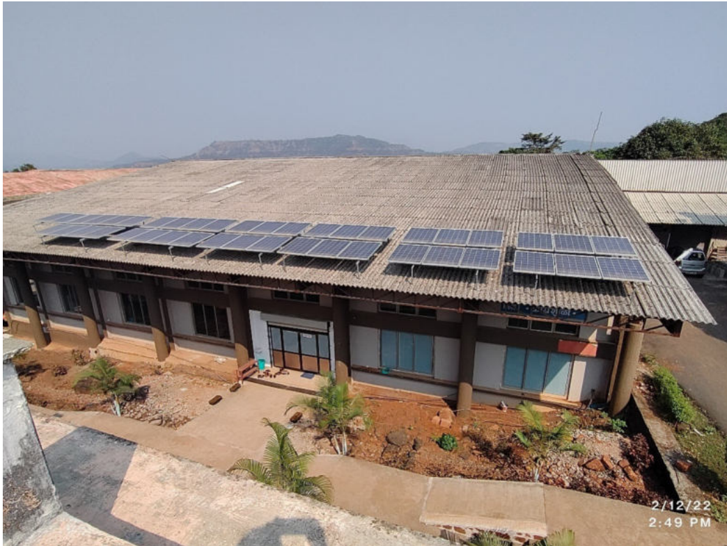
Workshop roof top
