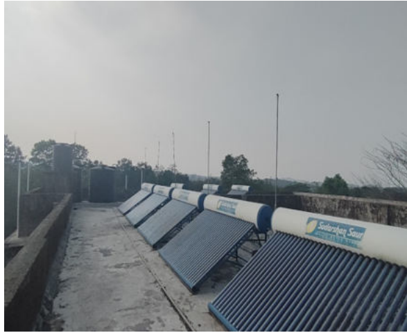
Solar water Heaterat hostel
