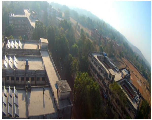
Solar water Heater at hostel
