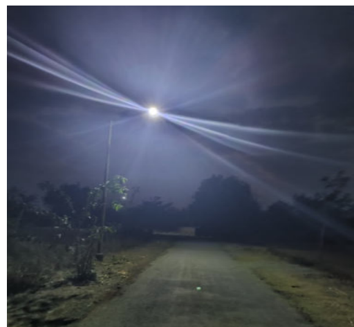
Solar Street light view
